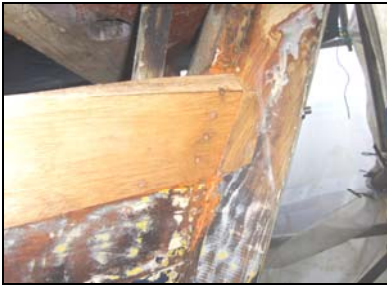
Cutting the joint for the next plank, note the long chamfer.
