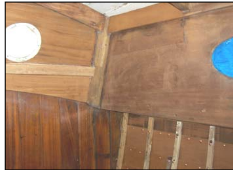
Detail of starboard cabin side replaced
