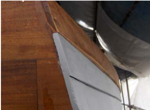
Planks still need some filling, but now all in place.
